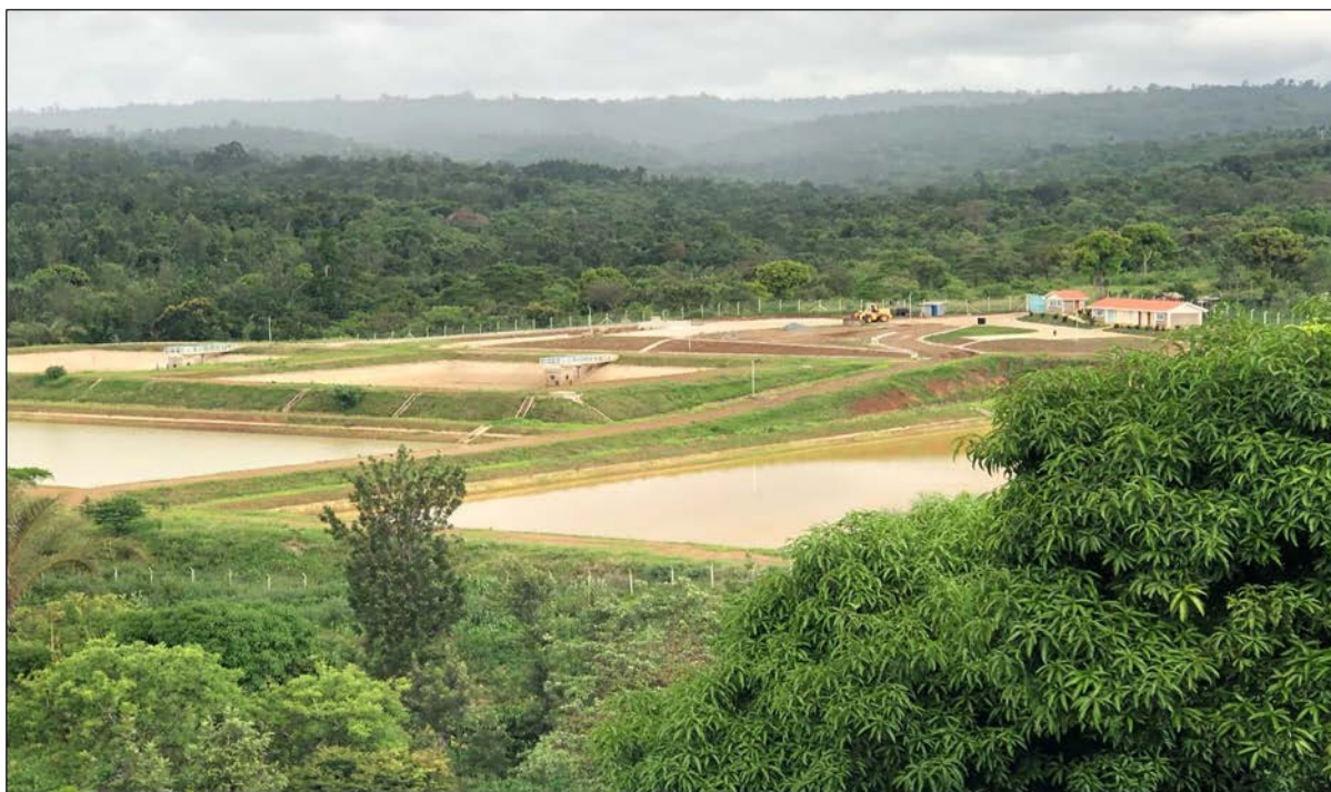
Plate 9.3:Chuka Treatment Plant.
