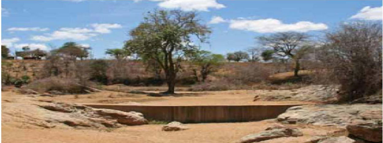
Plate 15.1: Typical Sand Storage Dam During The Dry Season (
