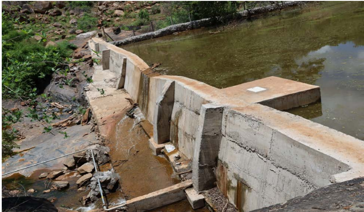
Plate 15.3: Kaiboche Earth Dam.
