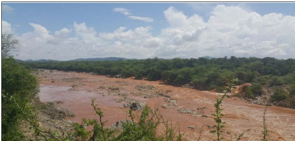
Plate 4.3: Tana River at Kibuka Falls, the Proposed Site for the Grand Falls Dam Project
